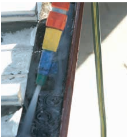
4) Spray the gutter & downpipes with water to soften and break up the dirt.
